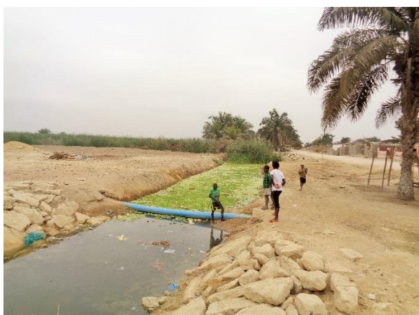
A drainage that had overflowed due to the piled up garbage in Catumbela, August 2015.
