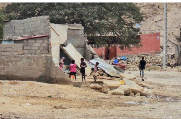
A house destroyed by the flood in Lobito, August 2015.
